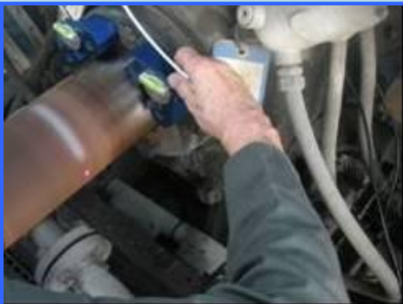
Figure 6. Removal Probe Mounts Attached to OB Bearing Housing of an ID Fan. Very Little Clearance is Needed to Install the Probe Mounts.
